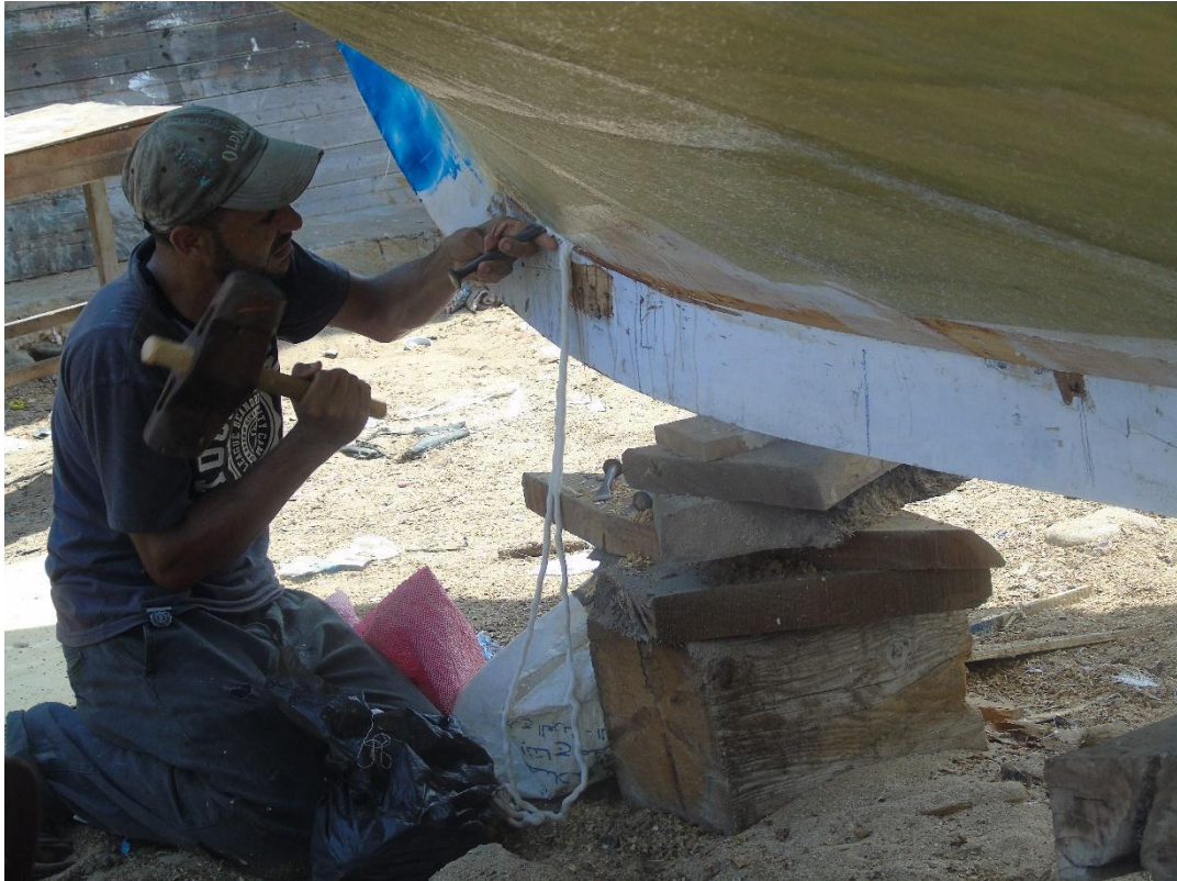
Fig.38: Caulking a yacht by a specialized labourer in Alexandria (© The author).
