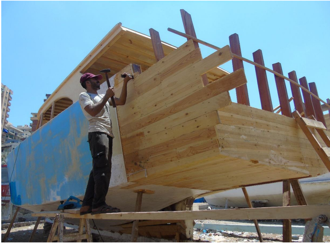
Fig.17: A labourer uses a hammer in the process of shipbuilding (© The author).
