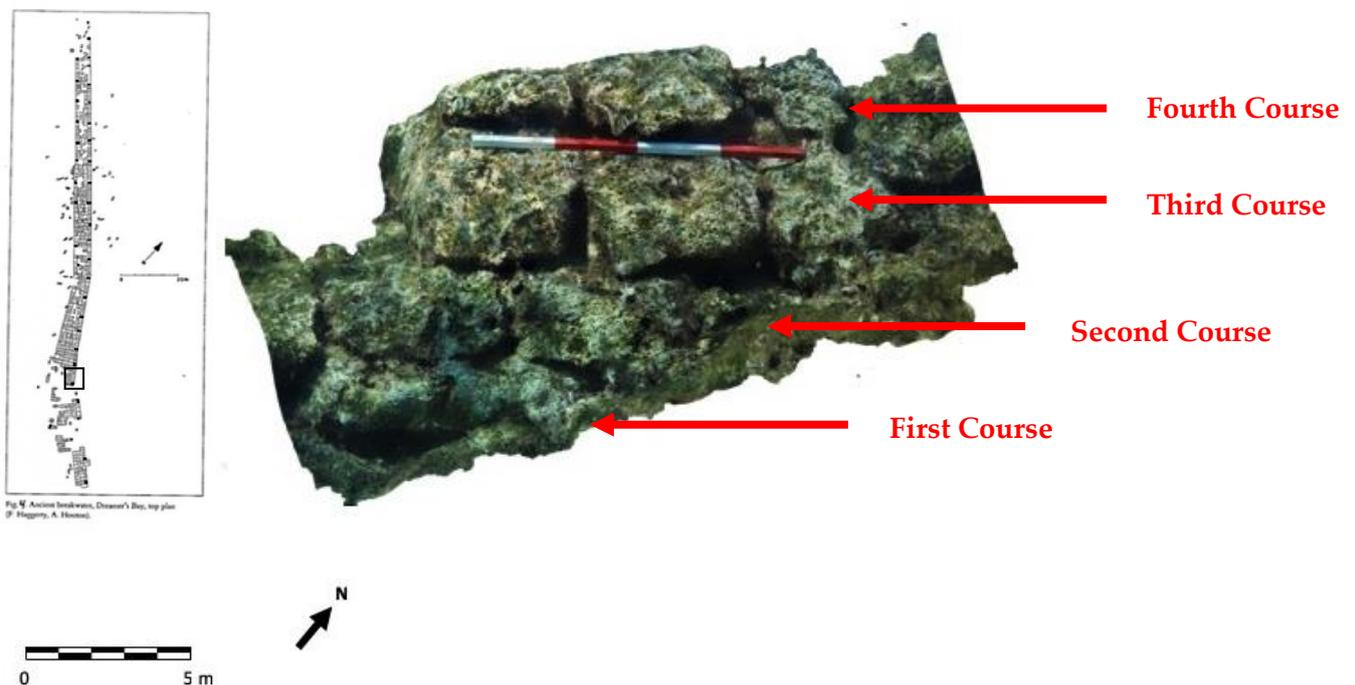
Figure 7: Orthophoto of the reconstructed portion of the eastern side of the breakwater (Photogrammetry survey and processing: M. Secci).
