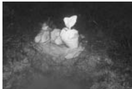
Covering Group 3 with sand and geotextile
