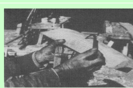
Fig. 2. Shipwright using hand callipers to take measurements off a 1/25 scale hull model that are used to construct full size master frames.
